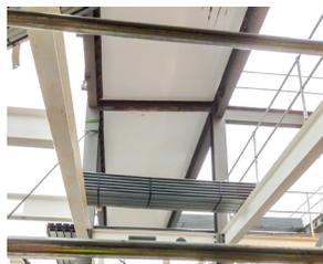
Intumescent paint was applied to the panels underside to achieve the required fire rating. Service runs were installed under the floors which was quick and easy to do.
