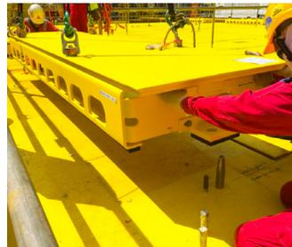
SPS plates and custom supporting frame are installed over a new or existing substructure. With welded or bolted connections the system is designed to absorb energy from dropped objects through plastic deformation of the plate and frame. These are custom designed to meet the requirements for each project and provide a useable working platform with immediate 100% load capacity.
