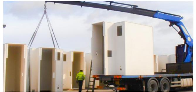
The first modular custody centres were built in Croydon for the Metropolitan Police. The flat panel system, delivered by truck, was quickly aligned and installed with the cell roofs forming a load bearing floor for the plant above.
