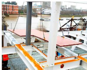
It allowed long spans. Its weight reduced the number of columns and beams required which increased building layout flexibility.
