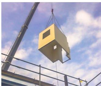
SPS enables contractors to rethink build sequences; to compress and accelerate even small build programmes. Modular SPS components can avoid the delays associated with building up complete floor by complete floor. With SPS, each bay can be built from the ground floor to the roof before proceeding to the next bay.
