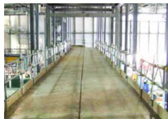
Large, open, suspended floor areas and walkway bridges benefit from the weight savings, fast installation and easier logistics of SPS. SPS panels permit longer spans with shallower and lighter beams. They are installed quickly and provide immediate 100% design load capacity.
