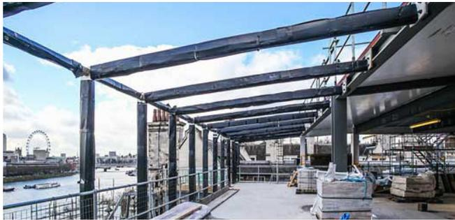
The use of SPS at 58 Victoria Embankment shows diversification in usage as it moves into the multi- storey building market. SPS panels were used on four of the seven floors, including the roof.
