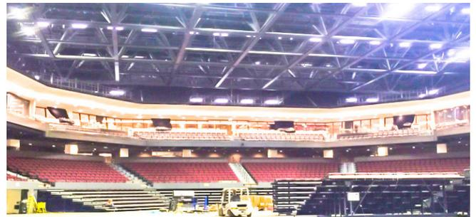
For China's first cinematically themed resort, SPS terrace units were used in the 3,000 seat main arena and a number of boutique small occupancy theatre units. The system's weight meant that it could be installed after the building had been completed, something that is not possible with other alternatives. SPS was able to overcome tight access issues and achieve the required performance and aesthetics criteria.
