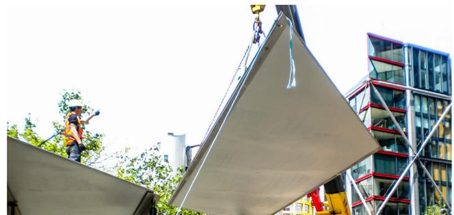
Located in one of London's most vibrant cultural destinations, Bankside Health Club was renovated to expand its studio offering. SPS was supplied for the gym's roof. The thin profile of the panels made them ideal for this modern structure. Delivered to site, with coatings applied, the eight roof panels were easily craned into position.
