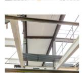
Intumescent paint was applied to the panels underside to achieve the required fire rating. Service runs were installed under the floors which was quick and easy to do.
