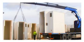
The first modular custody centres were built in Croydon for the Metropolitan Police. The flat panel system, delivered by truck, was quickly aligned and installed with the cell roofs forming a load bearing floor for the plant above.
