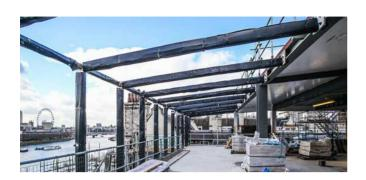
The use of SPS at 58 Victoria Embankment shows diversification in usage as it moves into the multi- storey building market. SPS panels were used on four of the seven floors, including the roof.
