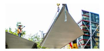
Located in one of London's most vibrant cultural destinations, Bankside Health Club was renovated to expand its studio offering. SPS was supplied for the gym's roof. The thin profile of the panels made them ideal for this modern structure. Delivered to site, with coatings applied, the eight roof panels were easily craned into position.
