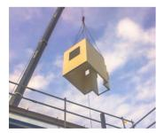
SPS enables contractors to rethink build sequences; to compress and accelerate even small build programmes. Modular SPS components can avoid the delays associated with building up complete floor by complete floor. With SPS, each bay can be built from the ground floor to the roof before proceeding to the next bay.
