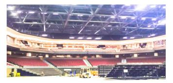
For China's first cinematically themed resort, SPS terrace units were used in the 3,000 seat main arena and a number of boutique small occupancy theatre units. The system's weight meant that it could be installed after the building had been completed, something that is not possible with other alternatives. SPS was able to overcome tight access issues and achieve the required performance and aesthetics criteria.
