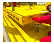
SPS plates and custom supporting frame are installed over a new or existing substructure. With welded or bolted connections the system is designed to absorb energy from dropped objects through plastic deformation of the plate and frame. These are custom designed to meet the requirements for each project and provide a useable working platform with immediate 100% load capacity.
