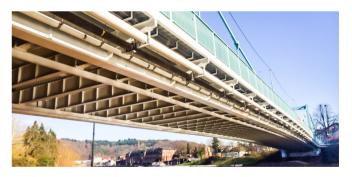
This suspension bridge, constructed in 1951, crosses the River Saar, Mettlach, Germany. Spanning 108m, the bridge has two lanes and was originally built with a steel-concrete composite deck. The bridge had its load carrying capacity reduced due to wear and corrosion but it was required to carry increased loads due to high traffic.
