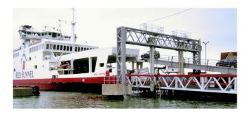
Red Funnel's East Cowes link-span bridge was reinstated and strengthened using SPS. The wearing layer was first removed after which the 36m long steel bridge deck was prepared. Perimeter bars were welded to the deck to create 35 cavities of 20mm depth. 8mm steel top plates, with factory applied wearing surface, were then welded to the perimeter bars to form air-tight cavities before the injection of the elastomer core. There was no disruption to scheduled services.
