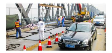
The orthotropic steel deck of this high volume road bridge in Zhaoqing Sihui City in Guangdong Province, China was suffering from fatigue. SPS was used to carry out a lane by lane strengthening and allowed the bridge to remain open to traffic throughout the project. Steel work and surface preparation was undertaken by a local contractor with IE undertaking the elastomer core injections. A total of 512sqm of bridge was reinstated during the Christmas to New Year period 2009.
