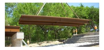
Texas DOT, supported by US Federal Highway Authority, used SPS panels to rapidly replace the deck of a remote two lane rural road bridge. The work took place over a weekend with no need for any concrete work. The SPS panels were delivered to site as half-width bridge modules integrated with longitudinal girders. The completed bridge comprised three 15m by 2m spans with expansion joints.
