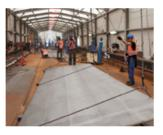
1.83m was added to its width using a total of 2,240m<sup>2</sup> of SPS panels. The bridge now accommodates four SPS strengthened vehicle lanes (two in each direction) and two newly installed tram lines; plus a two-way cycle lane and pedestrian walkways on either side which are accommodated on the newly installed SPS panels.
